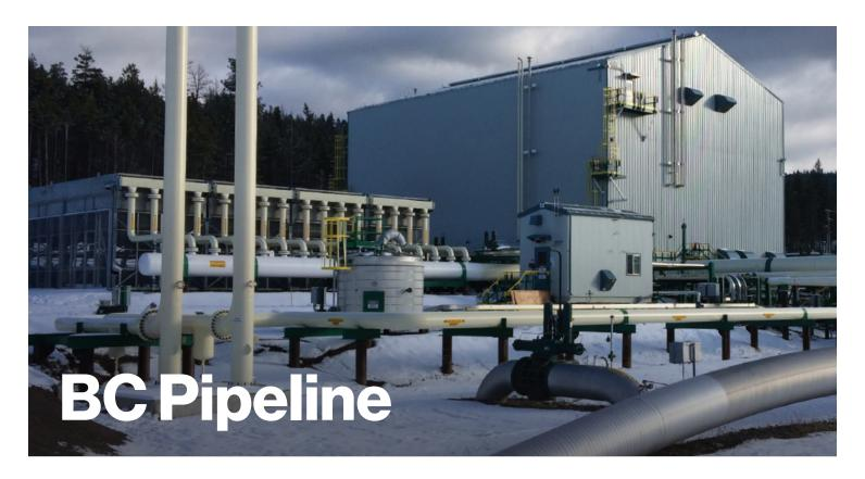
Enbridge's BC Pipeline, a natural gas transmission pipeline, is 2,953 kilometres (1,835 miles) long. It stretches from Fort Nelson, in northeast British Columbia (BC), and from Gordondale near the BC-Alberta border, south to the Canada-United States border at Huntingdon/Sumas.
